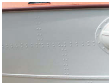
The rivets are small circles of paper 1.5 mm diameter, cut with a cookie cutter. These rivets are glued individually – there are more than 2,500
