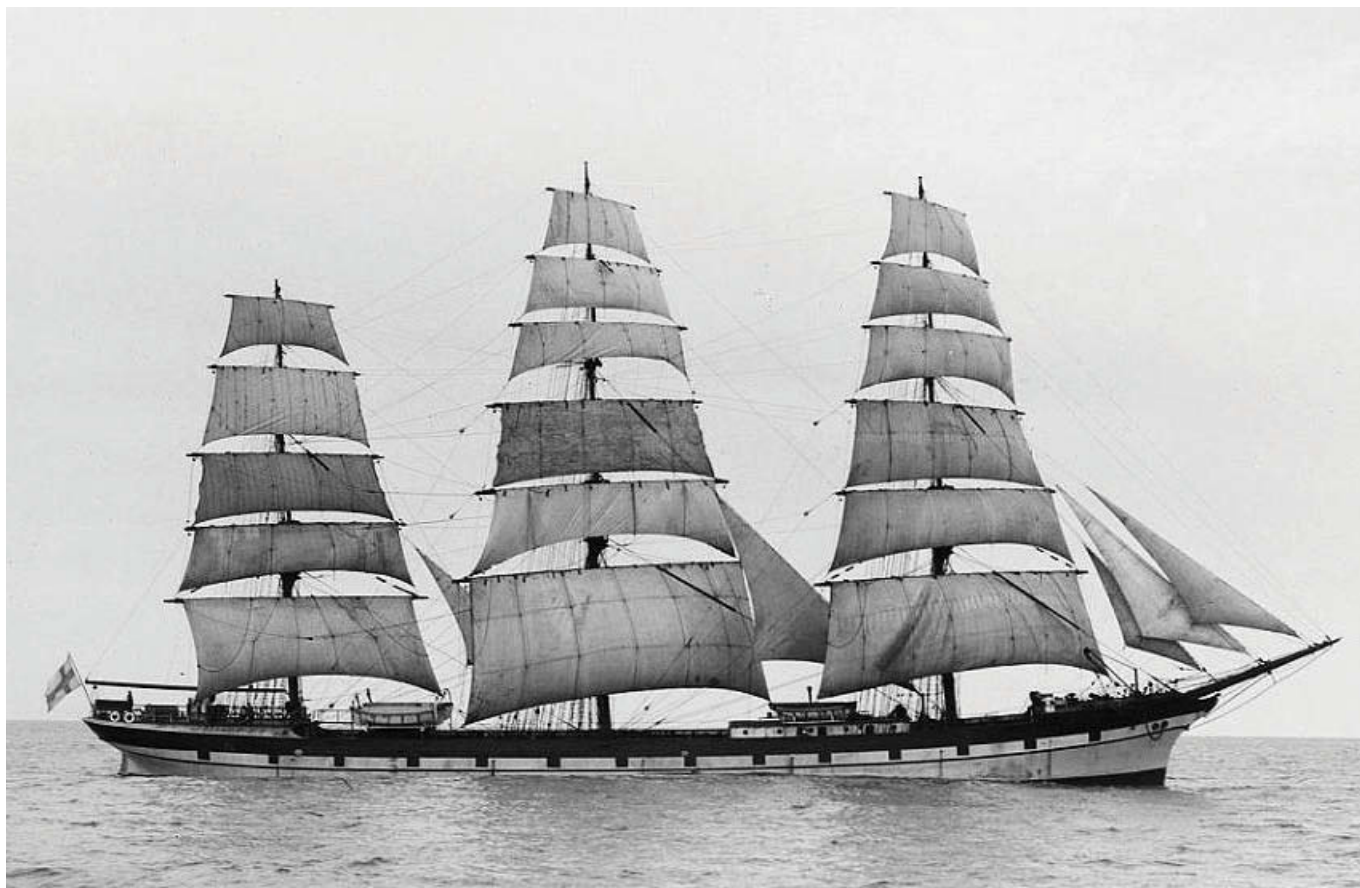
The last big full rigger to sail commercially, 'Grace Harwar'. She went to the breaker's yard in 1935, but is here seen in her prime, before WW1. Note that on this ship, the topgallants on the fore and main masts had been divided into upper and lower, only that on the mizzen was a single sail
