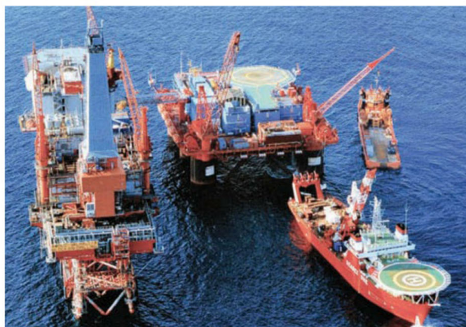
Seabex One attends this Amoco installation
