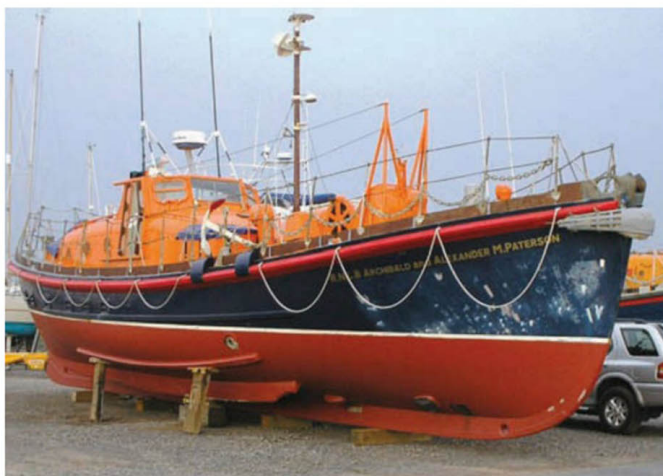
Andy's first ex-RNLI lifeboat, 'Archibald and Alexander M. Paterson' – a 52' Barnett Class, during restoration. Notice the work on the bow cross diagonal planking. The new anti-fouling coat is on – near to completion
