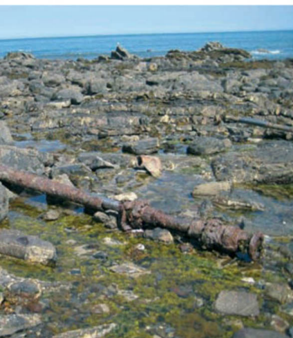
Outer shafts are eroded daily by the elements
