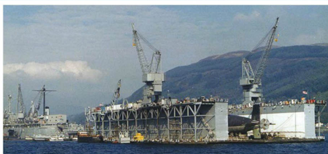
USS Los Alamos with new cranes, USS Simon Lake in the background
