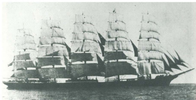
Preussen from the lee side, under all sail. Her enormous length to beam ratio is well seen from this angle. There must have been times when she was almost unmanageable, with that length, and all that sail
