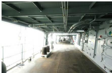
Port side passageway looking forward
