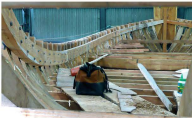
The deck beams nearing completion
