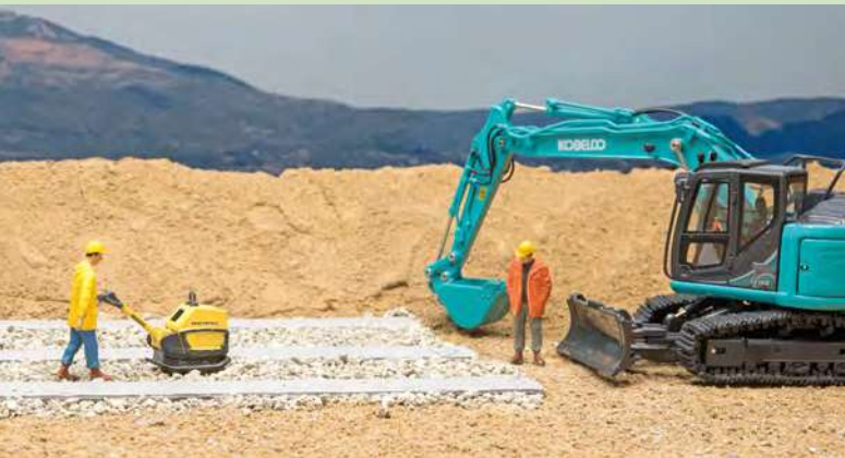
Preparing the foundation strips for the office container site.
