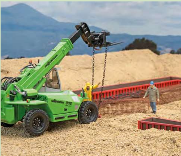
Installing the forms and re-bar for the shop foundations using a Sennebogen 305.
