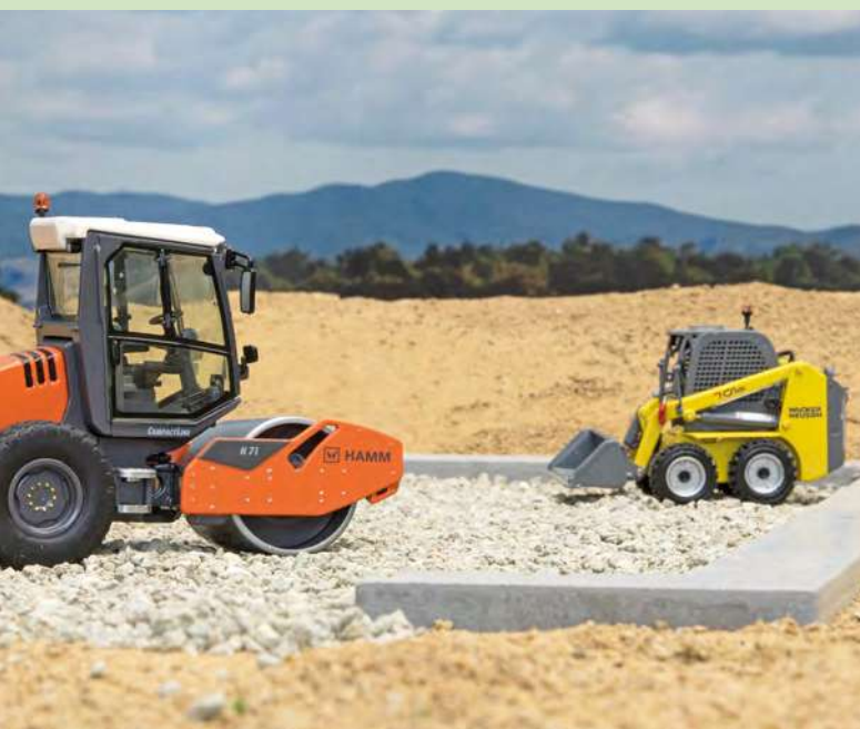
After the completion of the foundation, the subfloor is installed and compacted.
