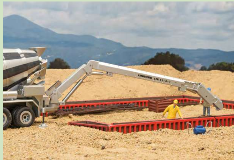
During the pouring of the concrete, a concrete mixer lorry with a conveyor belt is used.
