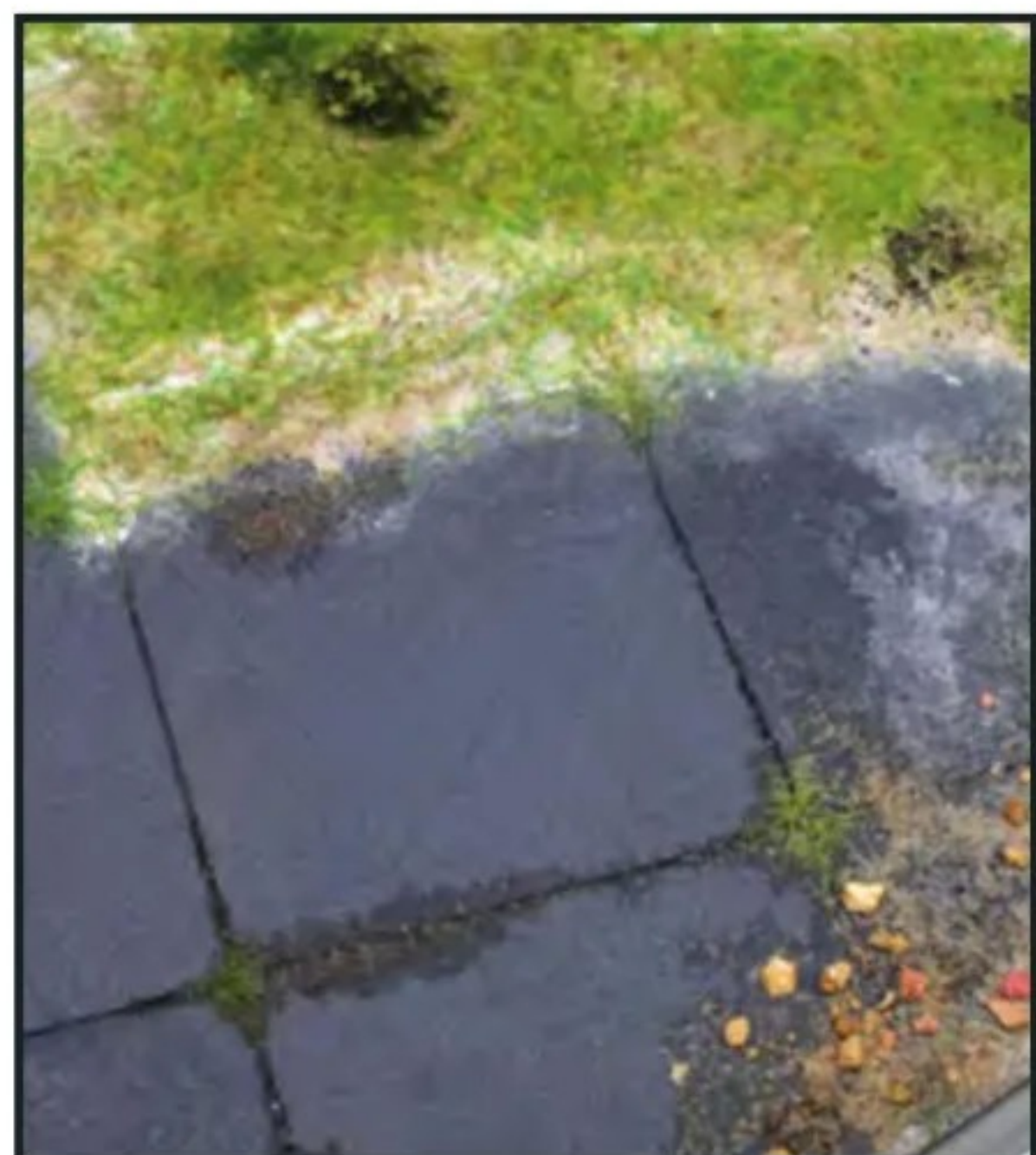
Close-up of the Styrofoam concrete pad. Once under paint, all of these disparate materials will start to come together
