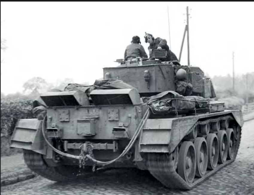
Comet 3rd RTR, Lubeck 2nd May, 1945. Again, we can see the double-bay 'Normandy cowl' over the exhaust; the centre slot allowing the barrel to be secured in its travel-lock on the rear deck
