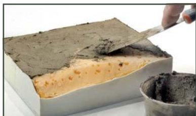
Over an expanded polystyrene foam base, the author spread a thin layer of tile adhesive, dyed in the mass with brown pigment powder
