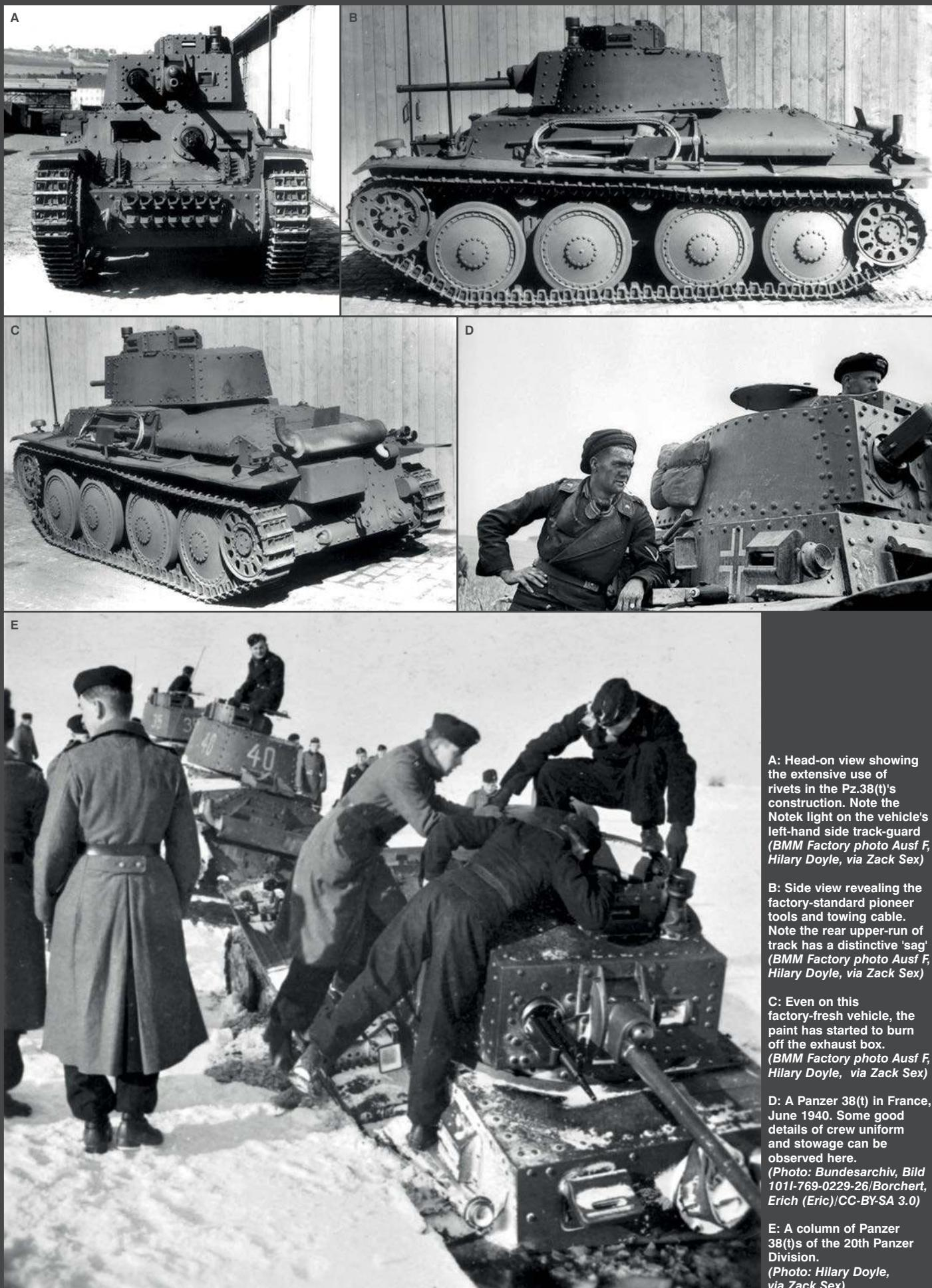
A: Head-on view showing the extensive use of rivets in the Pz.38(t)'s construction. Note the Notek light on the vehicle's left-hand side track-guard (BMM Factory photo Ausf F, Hilary Doyle, via Zack Sex)
