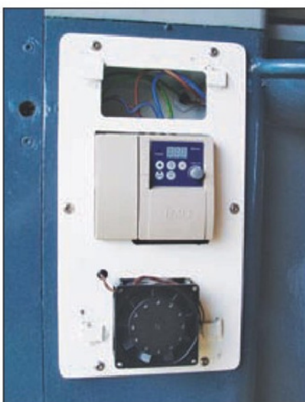
17. The inverter and cooling fan fitted.
