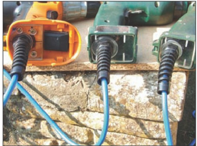
4. Strain relief bushes in place with cables installed.
