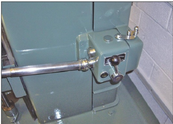
Photo 23. Gearbox and shaft refitted.
