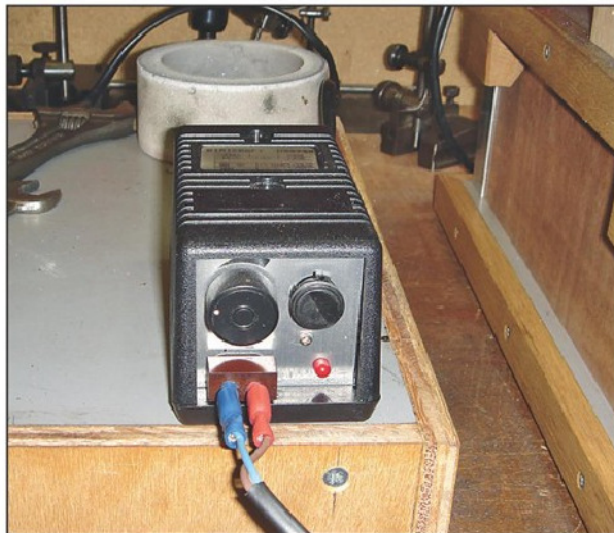
Photo 30. The transformer for driving the drill.
