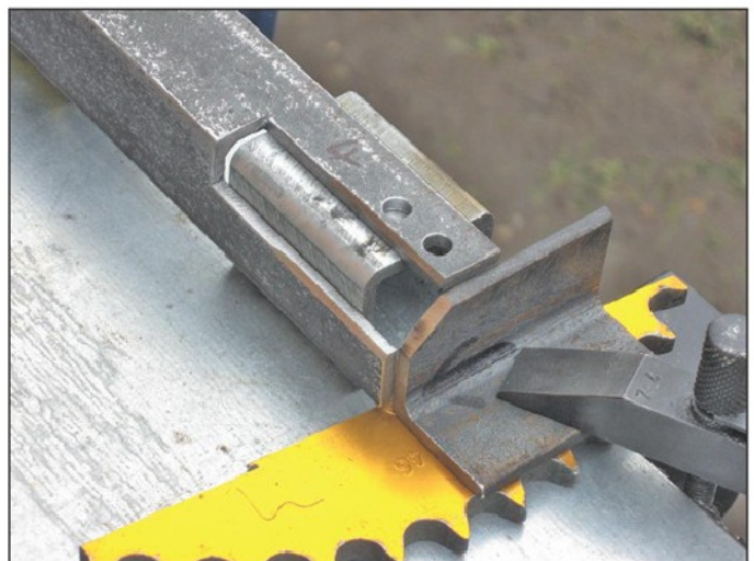
Photo 7. Aligning feet for welding.
