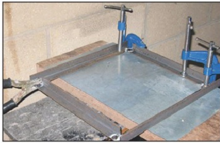
Photo 6. First frame side clamped ready for tack welding.
