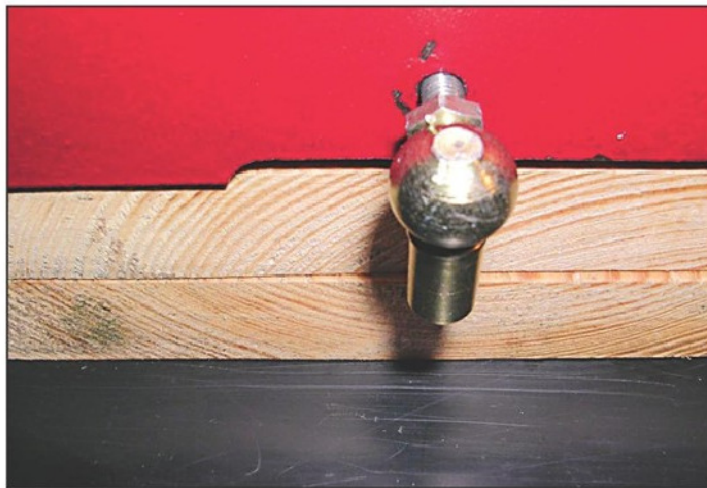
Photo 22. Bottom mounting hole for gas strut.
