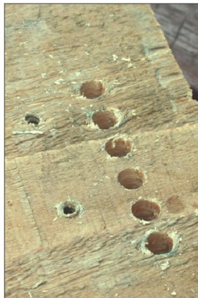
Photo 4. The first row of holes.
