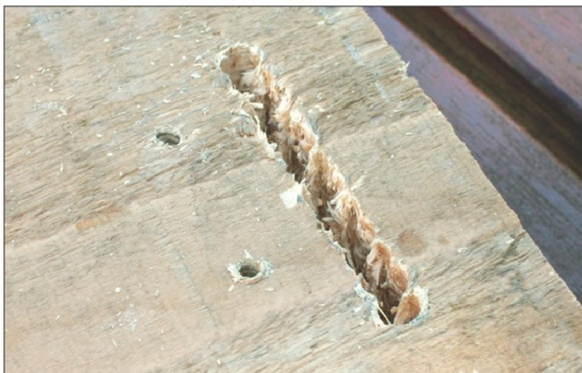
Photo 6. The second row of holes are drilled between the first holes.
