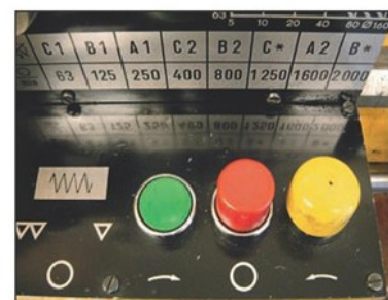
Photo 9. A cover is placed over the normal start position.
