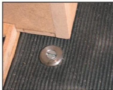
Photo 17 Flanged bush and countersunk screw used to secure matting.
