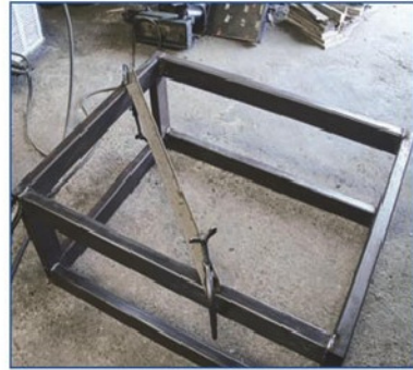
P13 Frame tack assembled, diagonal clamped to hold squareness
