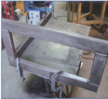
P12 End frame clamped vertically with first longitudinal added
