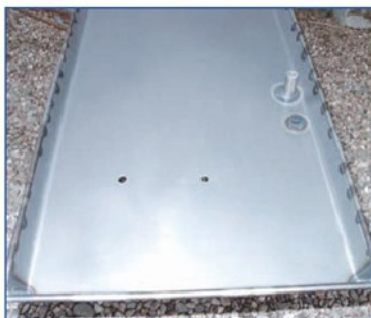
P06 Drip tray showing tubes welded along edges.
