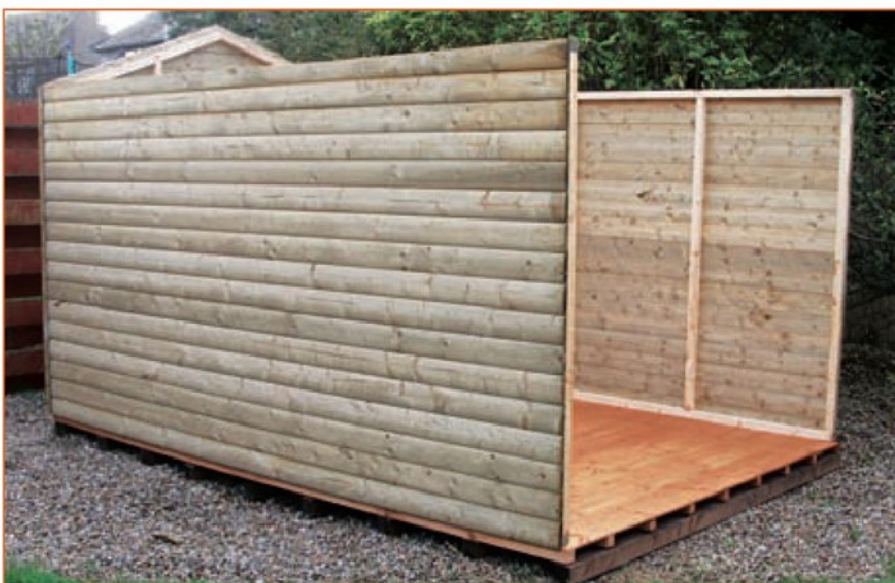
Photo 2 The shed partly erected.
