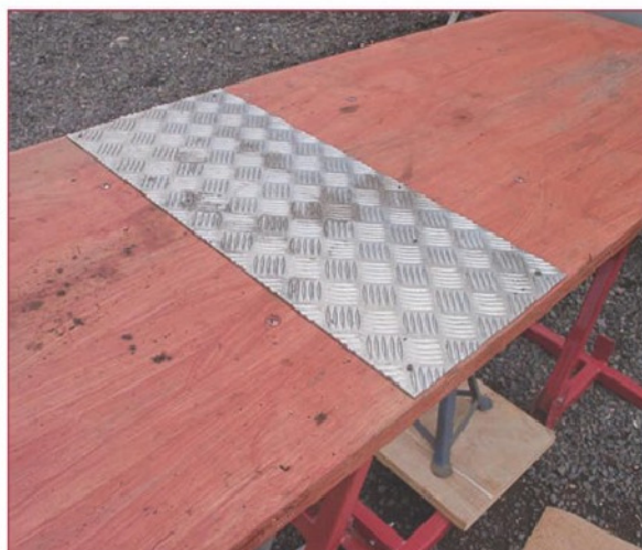
5. Tread plate stops centre stand digging into wood.
