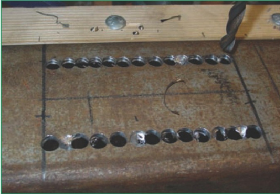
11. Slots in the base were formed by chain drilling-
