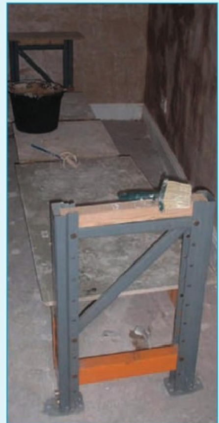
4. 'On site use for two end frames and two horizontal rails to give a 9in. lift by 10ft. long temporary platform for a plastering job
