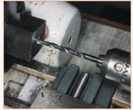
5. Opening up the hole in the block.
