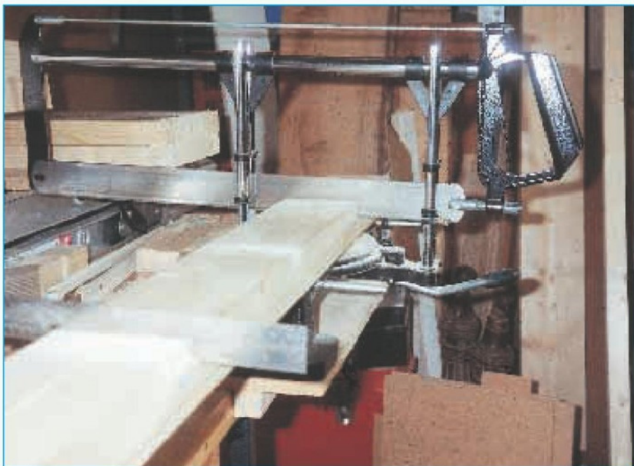
3. Using a mitre saw to cut halving joints in the verticals.
