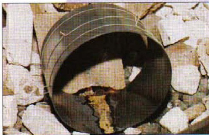
8. The rolled skirt is secured with iron wire while the brazing operation is carried out.
