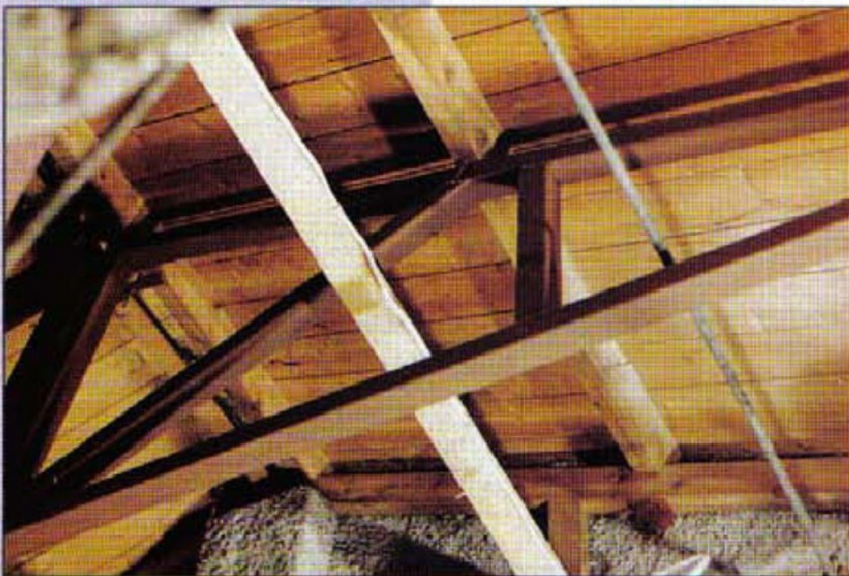
3. Strengthening a roof structure was quick and easy using the MMA welder. Trusses were assembled in situ using 50mm x 50mm box section steel, making it easy to match the steel sections to the existing structure. During the assembly, there never was a requirement to lift or hold anything heavier than one length of the box section.
