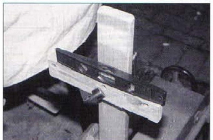
8. Setting timber piece level side-to-side
