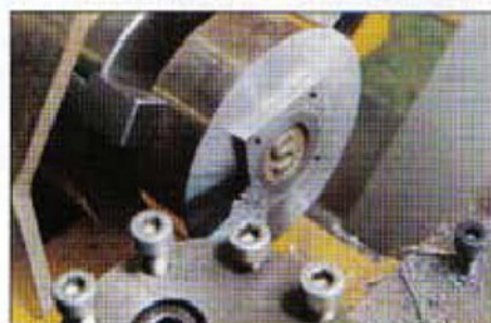
16. Using a plain disc faceplate, machined in situ, to face the valve chest cover. Thin film double adhesive being used to hold the cover.
