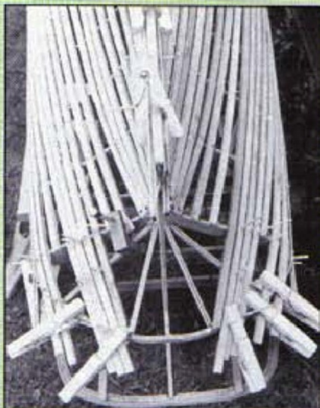
Planking begins to form the moulding surface.
