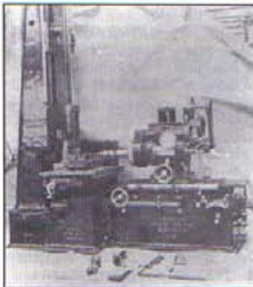
Fig. 22: Churchill pendulum grinder working on curved expansion links, c. 1930.
