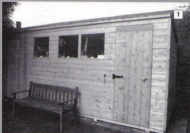
1: An off the shelf garden shed, can be transformed. Attention to detail in the treatment of exposed surfaces, insulation and heating have made this into a comfortable and airy working environment.
