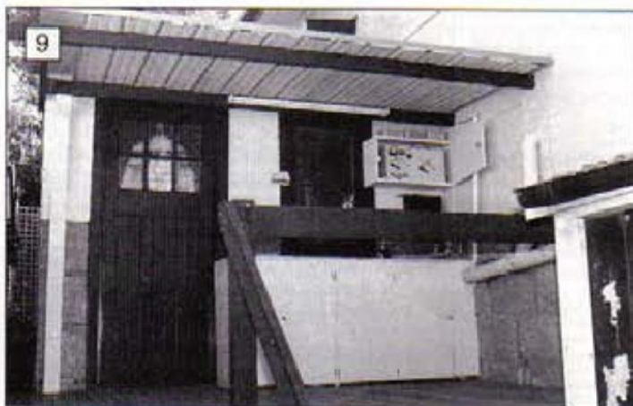
9: Part roofed rear deck. Bench with sink. Cupboard with electroplating current source.
