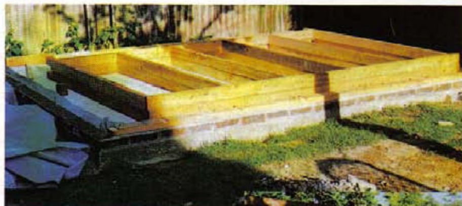
Trial assembly of the side frames.
