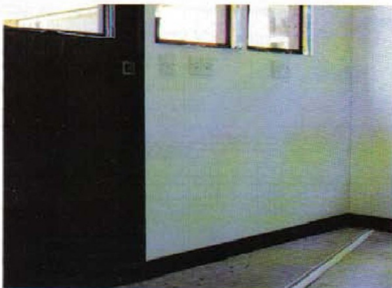
Skirting boards in place. Painting and staining finished.
