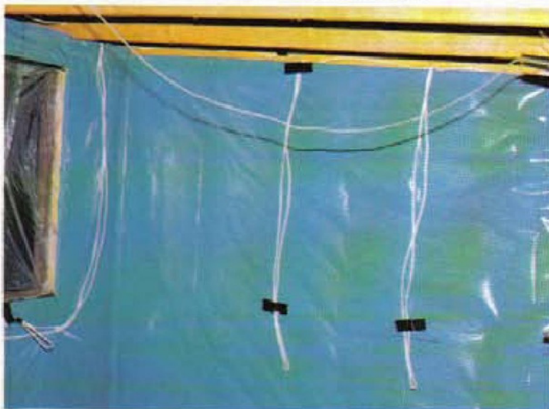
Wiring in position.
