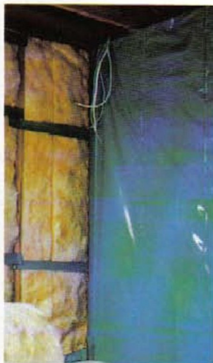
Damp proof membrane fitted over insulation.
