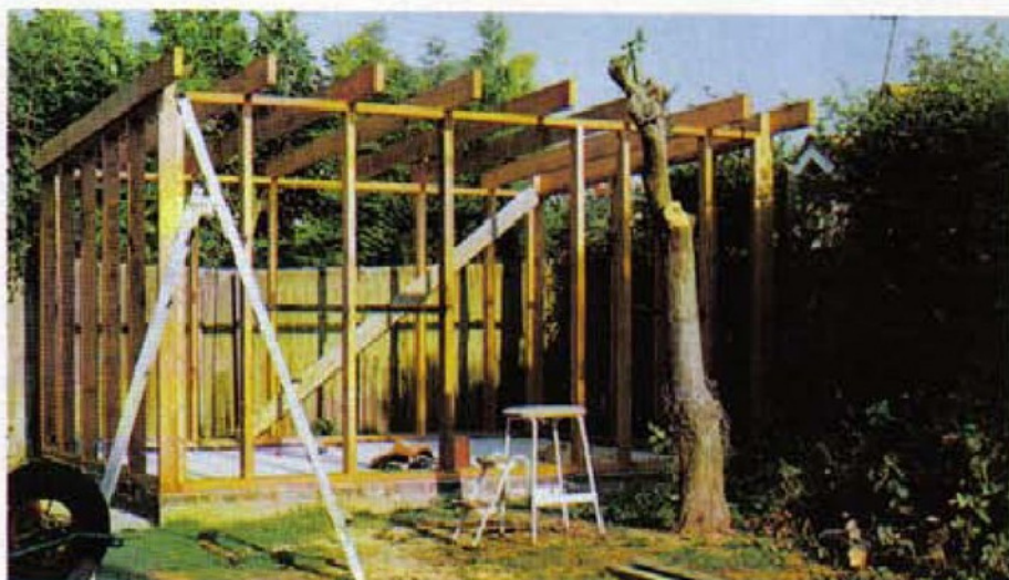
Above: Assembled frames taking the strain! Below: Frame with rafters in place.
