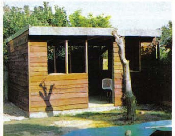
Nailing cladding over breather paper. Roofing felt completed. Most of the cladding finished.
