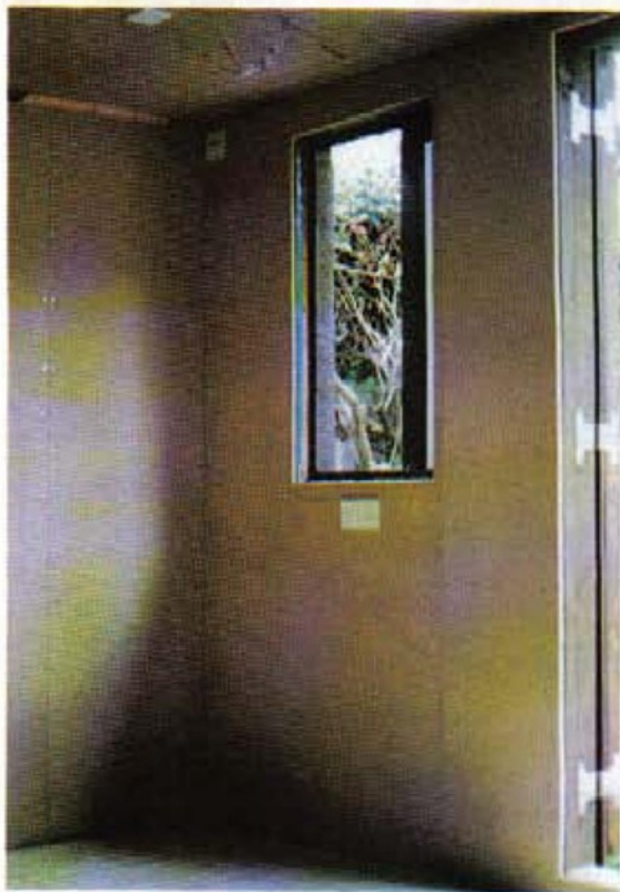
Interior panels complete.
