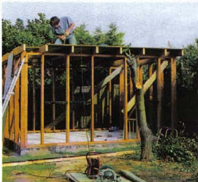
Screwing T & G roof panels in place.
