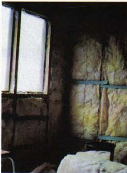
Rockwool insulation held in place with paper strips.
