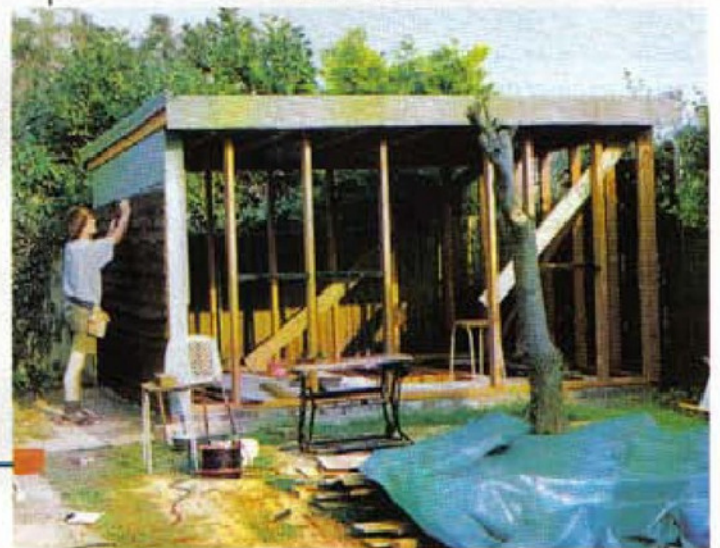
Nailing cladding over breather paper. Roofing felt completed. Most of the cladding finished.
