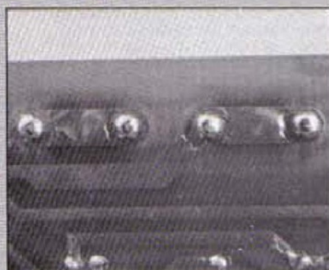
Left hand pair of joints were de-soldered using the wick, right hand pair the sucker.
