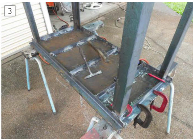
Welding steel angle support rails under the bench top.
