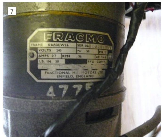
Label on the single phase worm geared motor.
