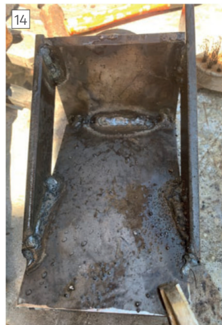
14 Final results of the welding. Not at all the prettiest welding and not improved by forgetting to use my can of anti-spatter at times. Penetration achieved however and I doubt it will fall apart in use!
