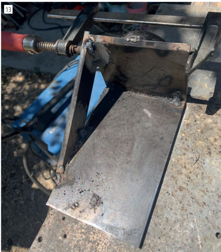
13 Tack welding the first of the two side braces. The tack welds on the main to end plates can be seen as well
