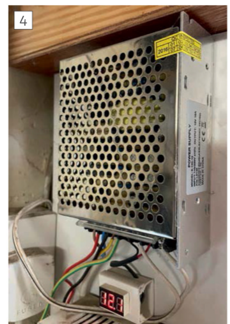
Test of uncased 12V DC power supply before fitting of an outer enclosure and securing of cables.
