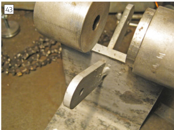
43 Bracket after welding
