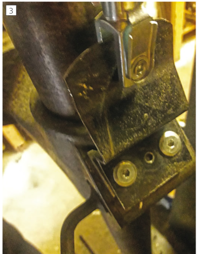
The yoke for the counterweight anchor.
