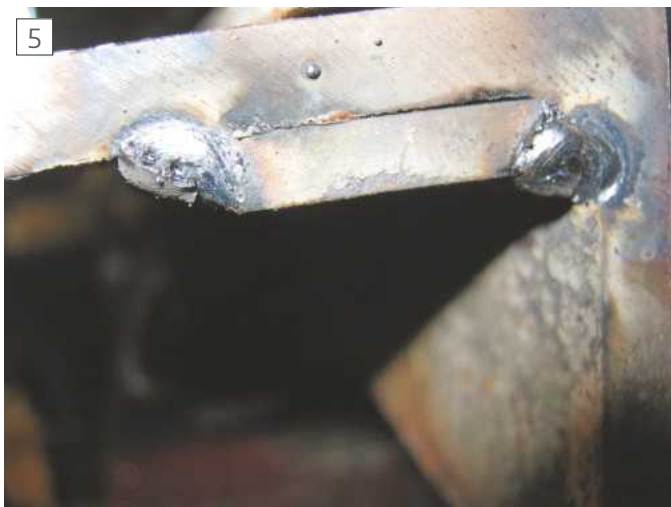
Additional backing pieces for screw after welding.
