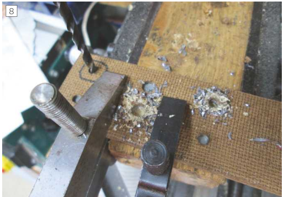
Utilising the template to drill the holes in the temporary support plate
