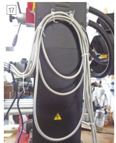
DRO, excess cable looping.
