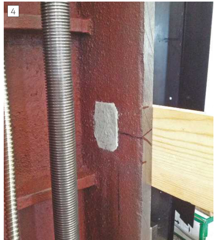
Z-axis, completed mounting pad.
