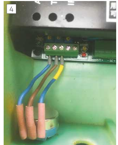
Installing the Potentiometer
