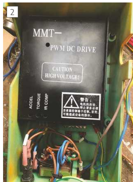
The Controller Installed
