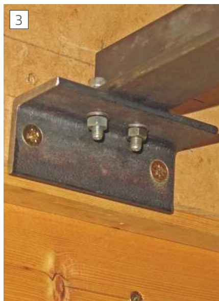
Wall end support.
