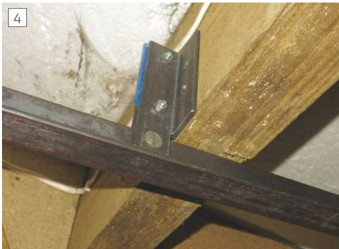
Hanger from beam.
