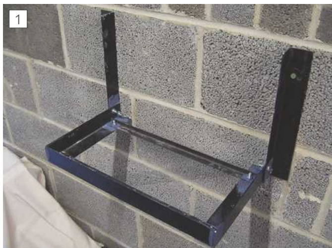
The finished and installed frame
