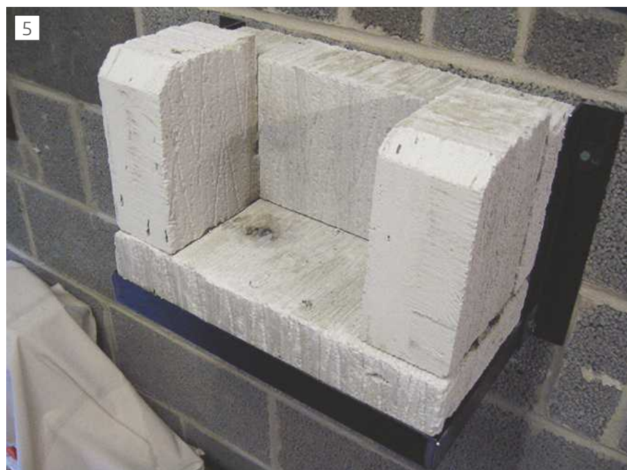
The finished Brazing Hearth
