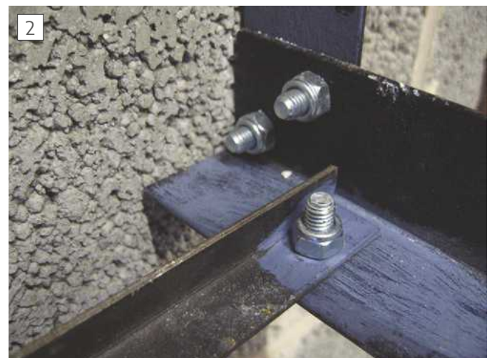
Non-rotatable bolted connection
