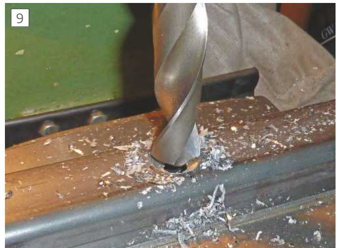
Enlarging hole in box section
