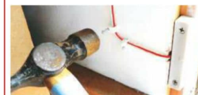
3 Pin the siren and contact wires in place with clips provided
