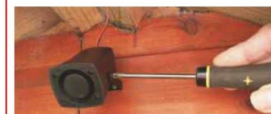
2 Fit the siren to the exterior, high up and out of reach
