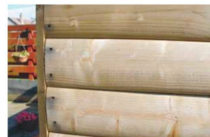
Photo 4: Log lap construction.
