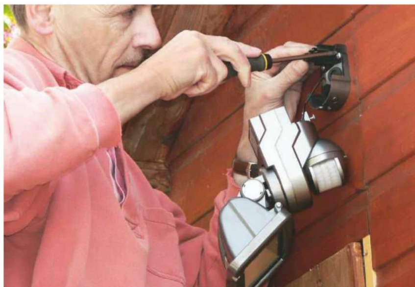
Fitting a PIR light
