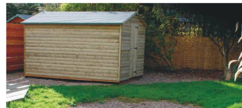
Photo 7: The finished shed. This one is 8ft. X 12ft.
