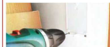
1 Drill the wall to mount the backing plate of the control panel
