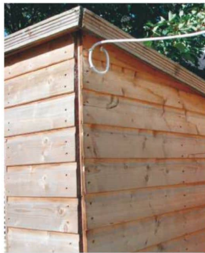
Photo 2: A pent roof.
