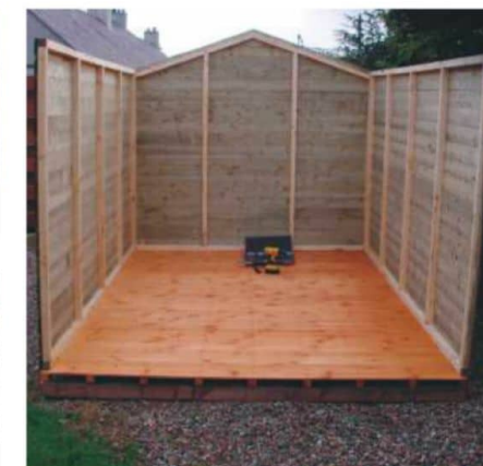
Photo 9: The shed partially erected.
