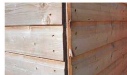
Photo 3: Tongued and grooved construction.
