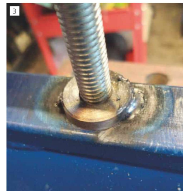
Drilling ex Locating Washers tack welded in place. haust passage.
