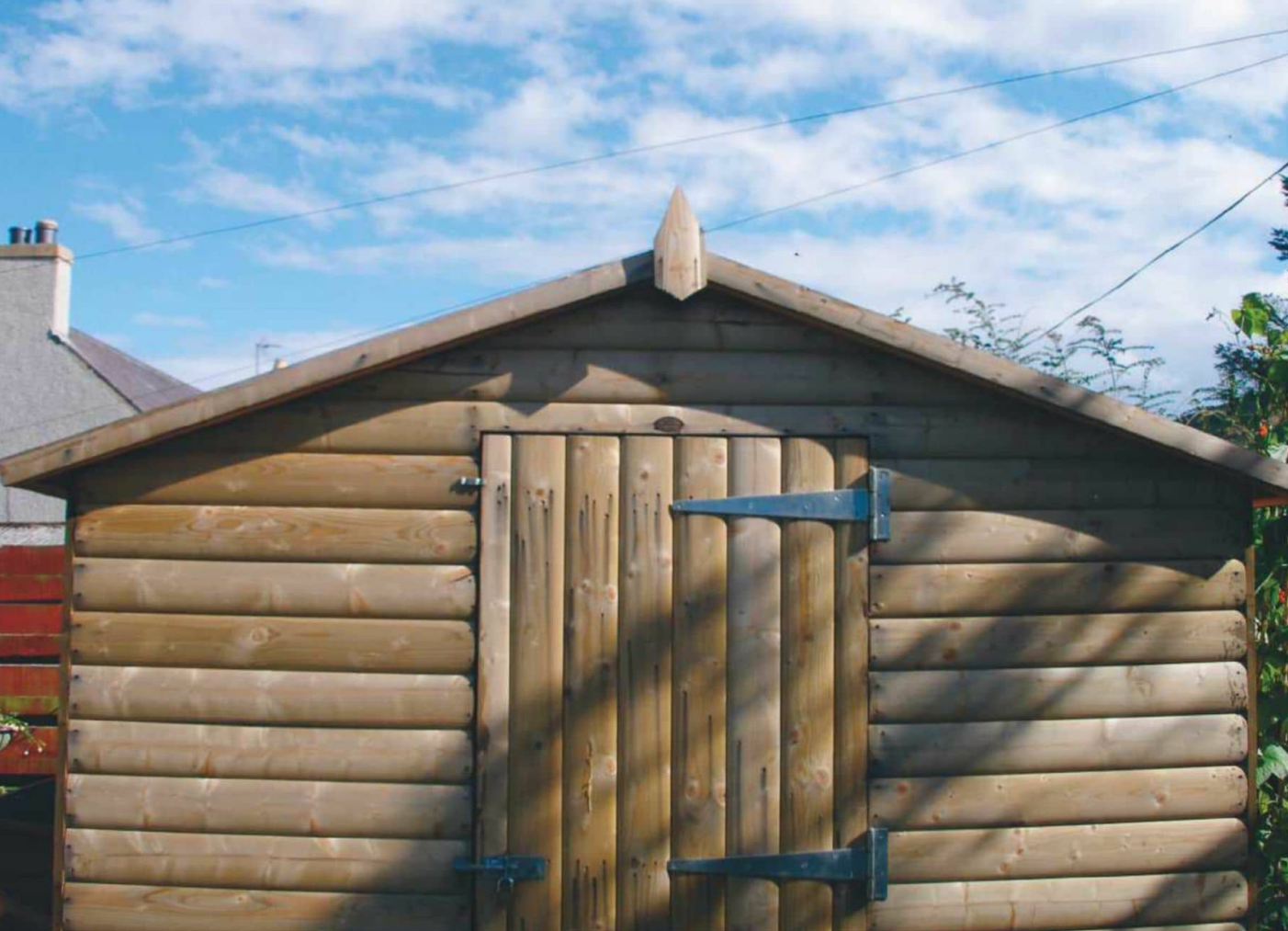
Photo 1: An apex roof
