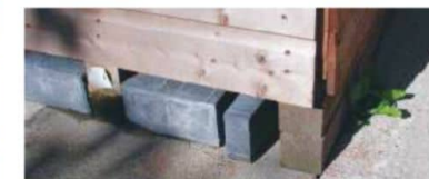
Photo 8: Fence posts under the shed. The bricks are to stop the dog getting under.
