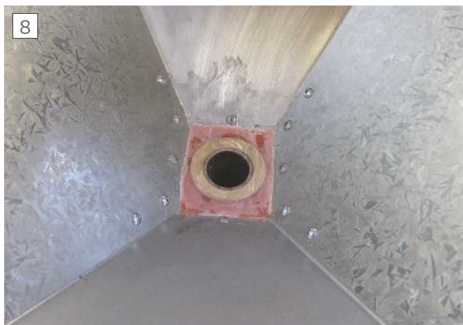
1½ inch dia. flanged collector resin bonded into the bottom of the hopper
