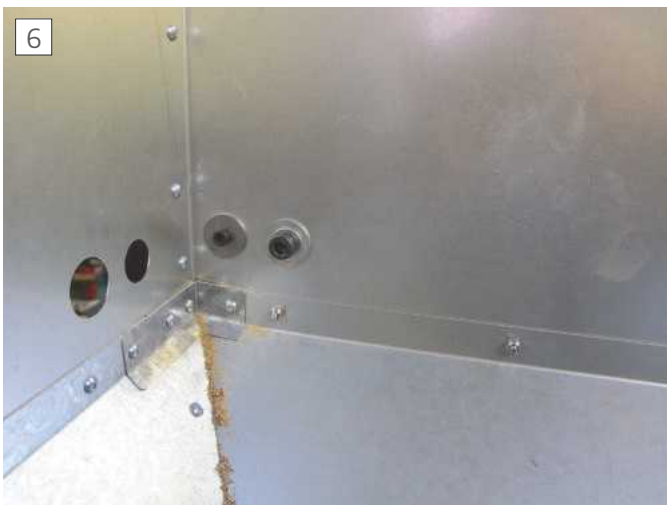
M6. screws with large diameter washers for securing hole cutting buttons.
