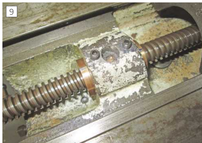
The two halves of the new table feed nut in place fixed with grub screws
