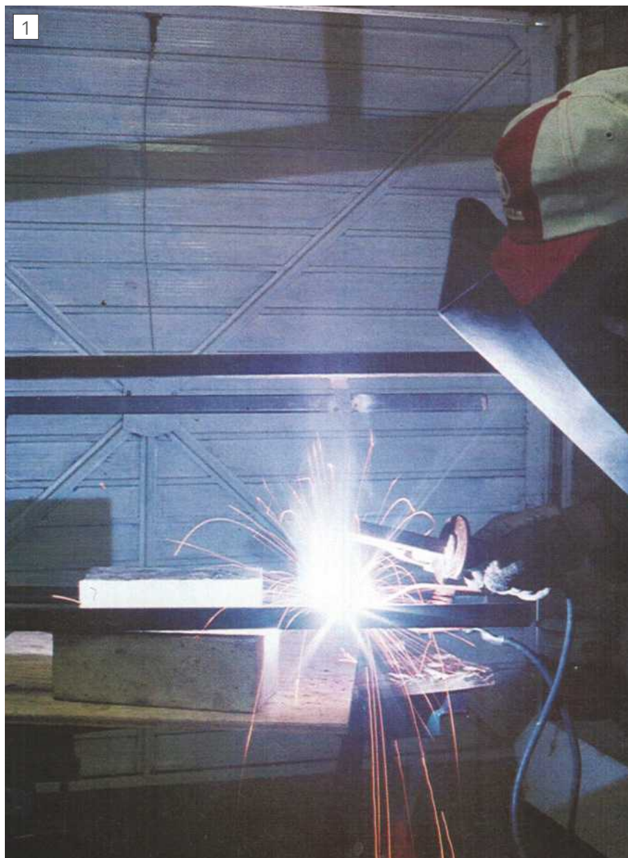
Arc welding in progress, note the use of protective gear.
